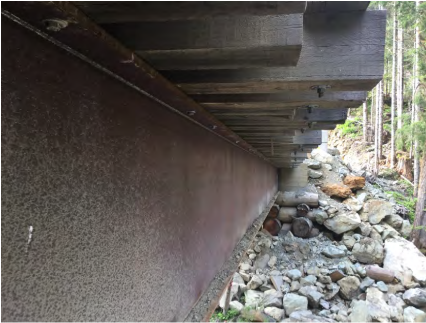
Deck panels bolted to ties
