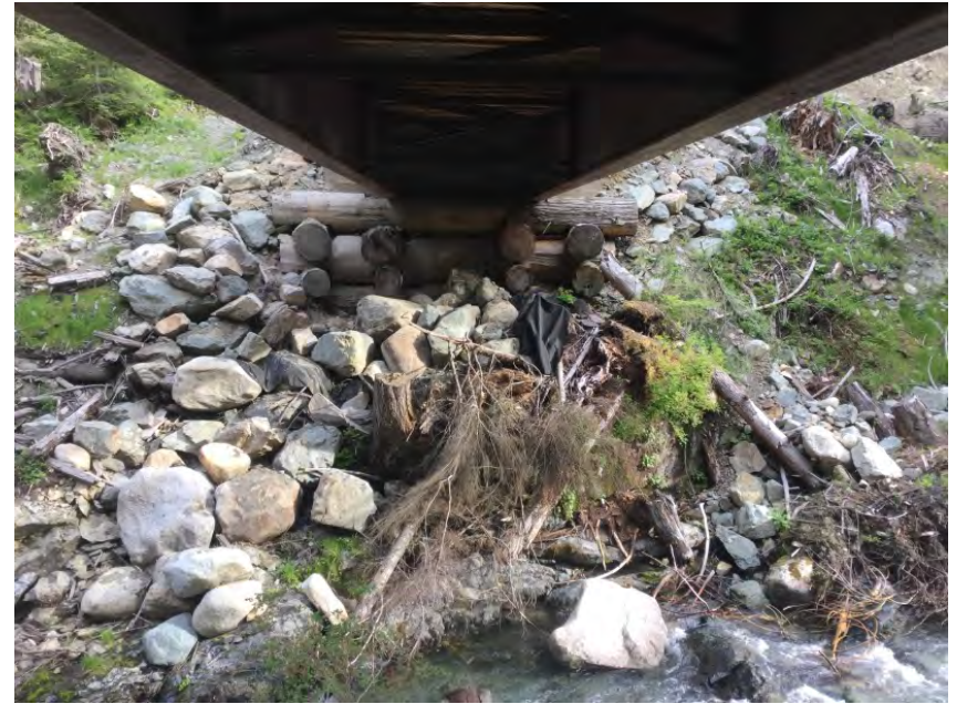
Right Bank Abutment when facing downstream
