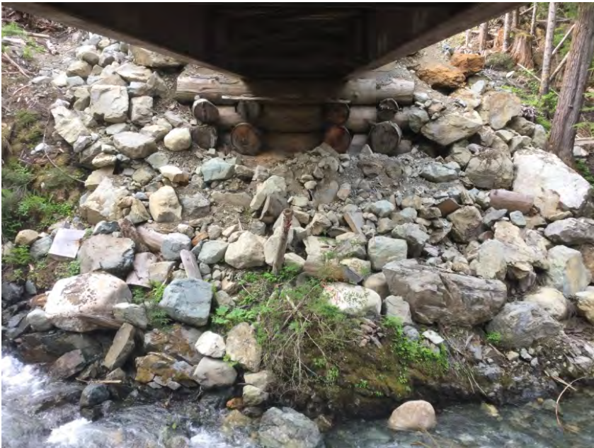
Left Bank Abutment when facing downstream
